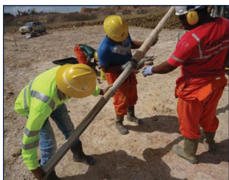
FIGURE 7. Full core recovery: sonic drilled in bauxite (Surinam).
